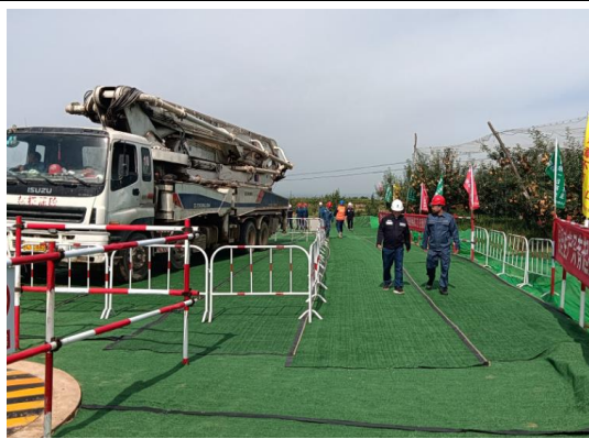
N0735 塔基区临时苫盖
