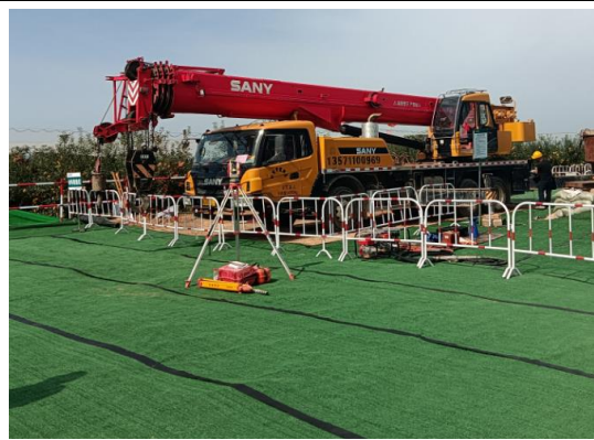
N0735 塔基区硬质围栏
