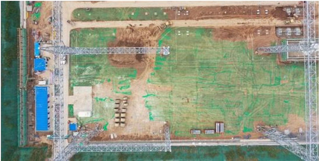
裸露地表临时苫盖 (2020.11)
