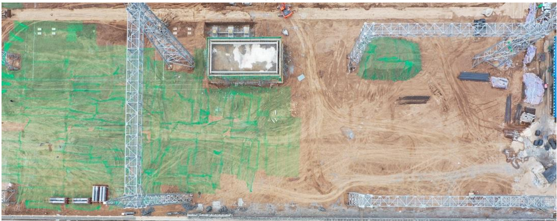
临时堆土密目网苫盖 (2020.11)
