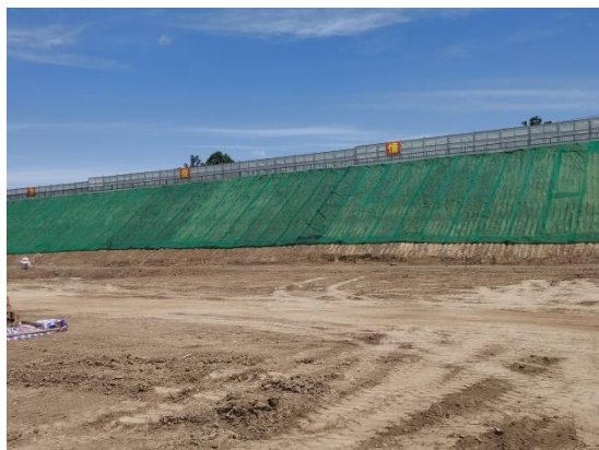
边坡临时苫盖 (2020.5)
