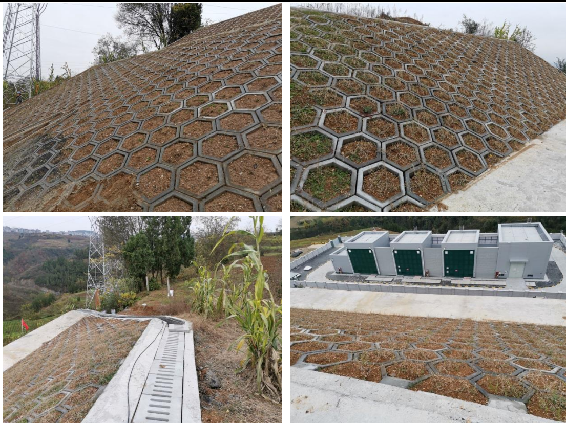
护坡植草砖及撒播草籽
